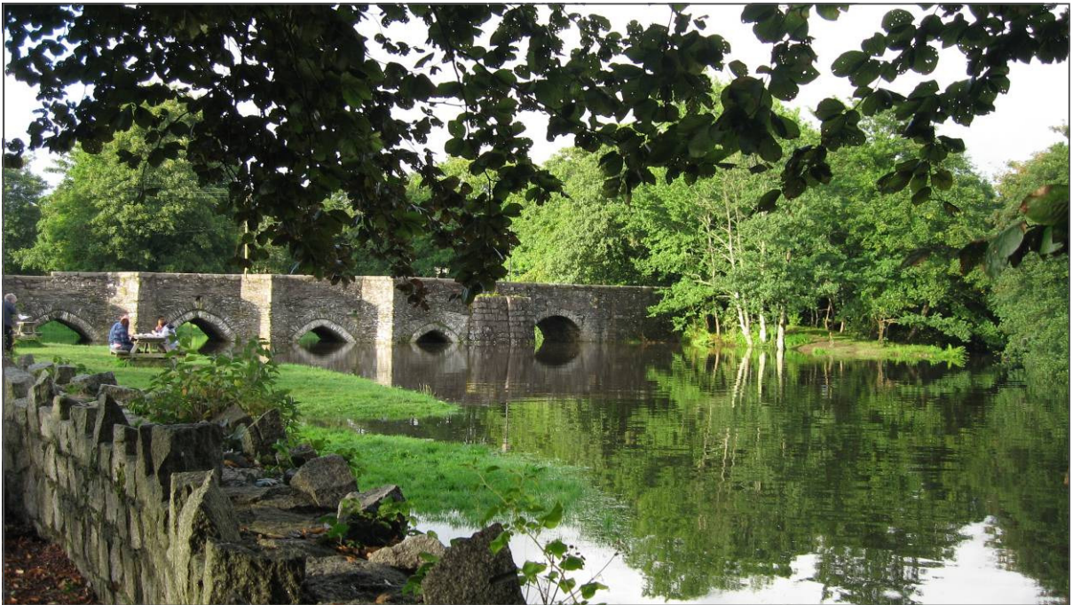
Lostwithiel Bridge at High Spring Tide
