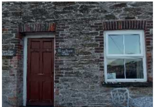
Stone front and brick arches
