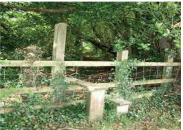
Stile in tree tunnel at Colquite
