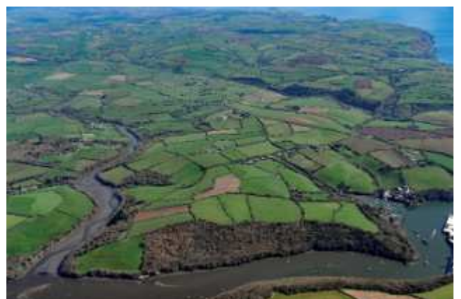
The AONB area with Penmarlam in right hand corner
