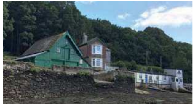
Waterside boathouses etc. at Mixtow
