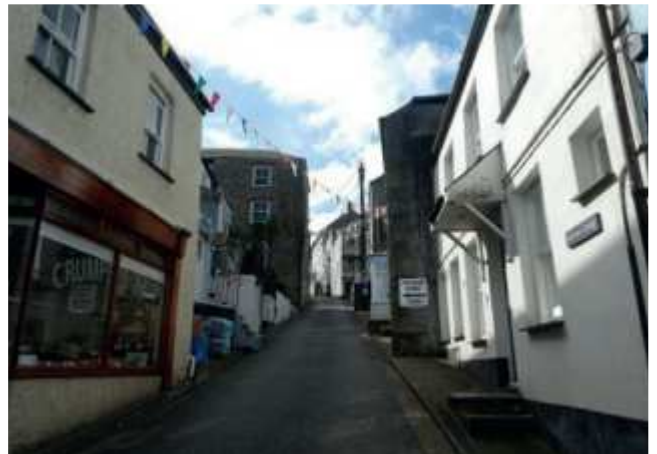
Fore Street looking uphill
