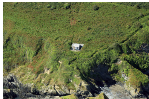
Above: Lantivet watch house, with steps down into cove; below: rock-cut steps in Palace Cove.
