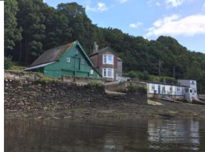
Waterside boathouses etc at Mixtow
